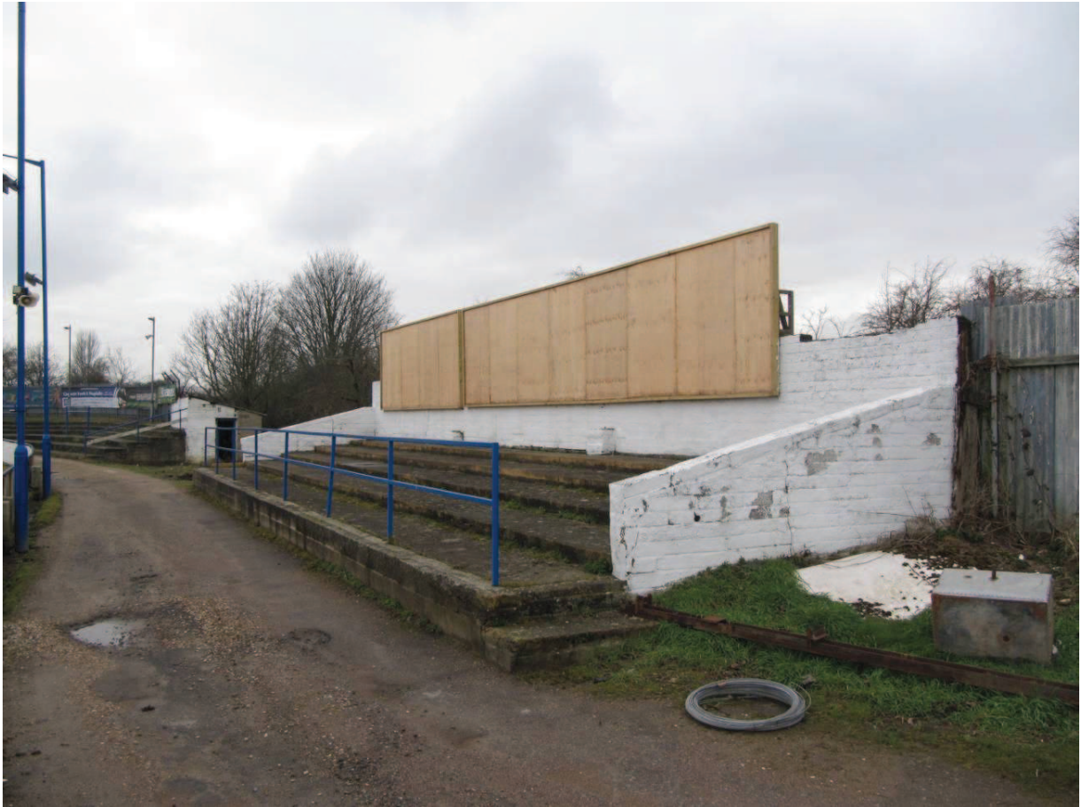
Photograph 16 – terrace to north side of stadium
