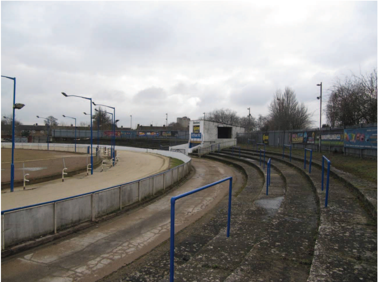
Photograph 19 – terraces to west side of stadium
