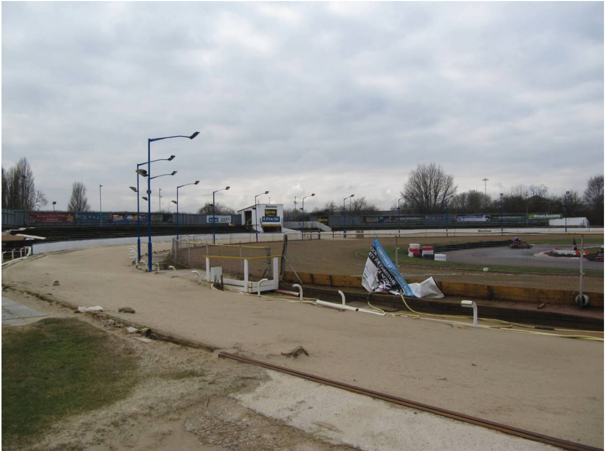
Photograph 17 – terraces to west side of stadium
