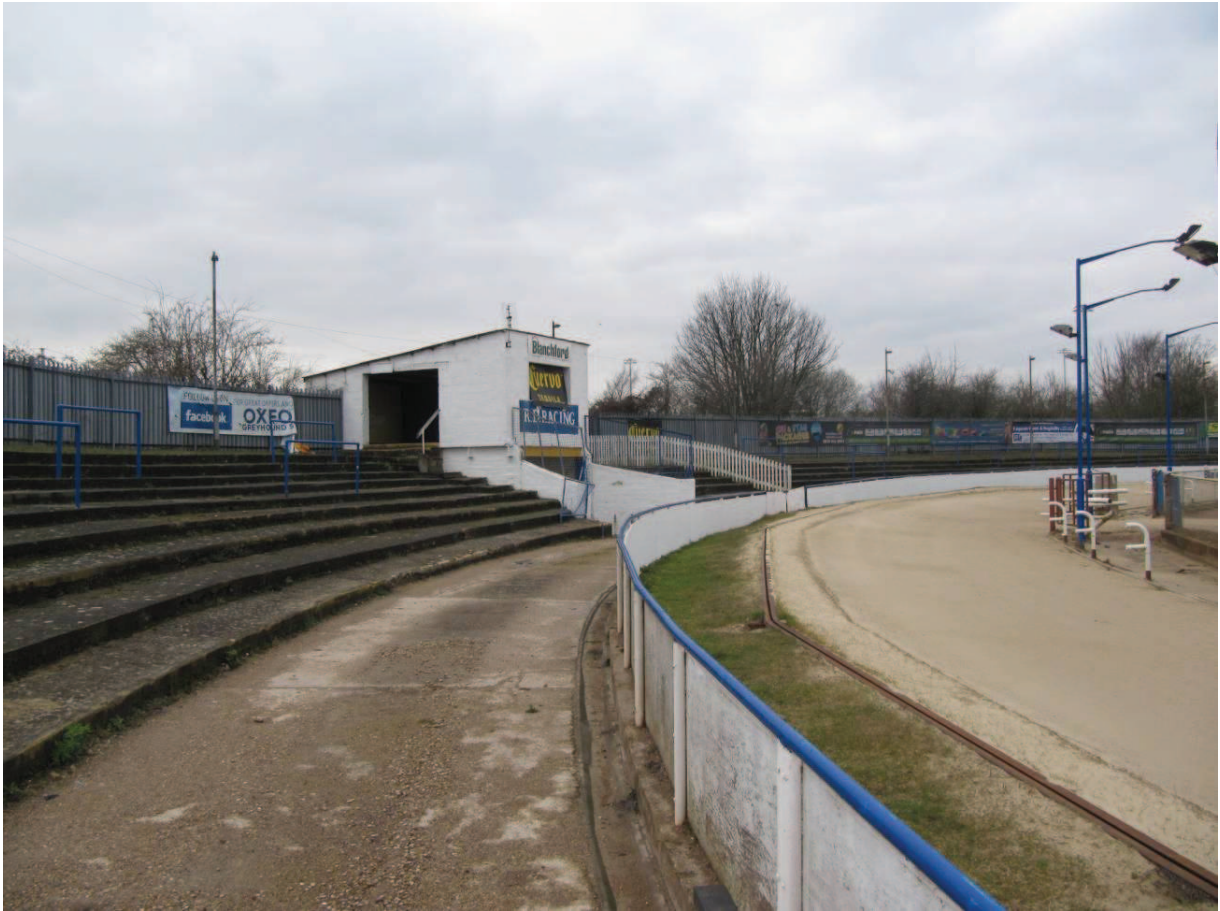
Photograph 18 – terraces to west side of stadium
