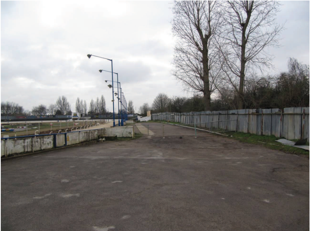
Photograph 15 – north side of stadium
