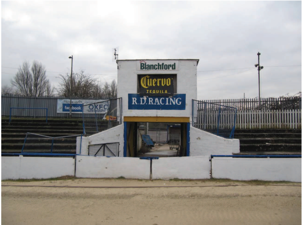
Photograph 20 – terraces to west side of stadium
