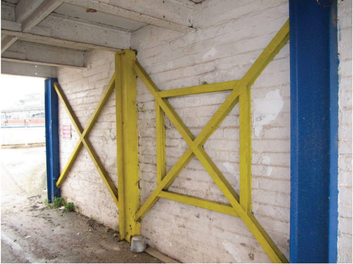
Photograph 23 – entrance to yard area to west side of stadium
