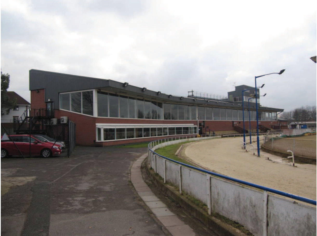
Photograph 3 – front of main stand
