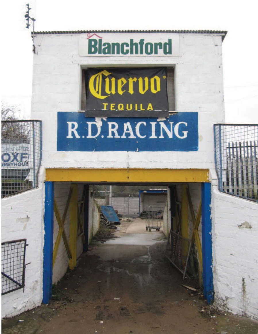
Photograph 22 – entrance to yard area to west side of stadium
