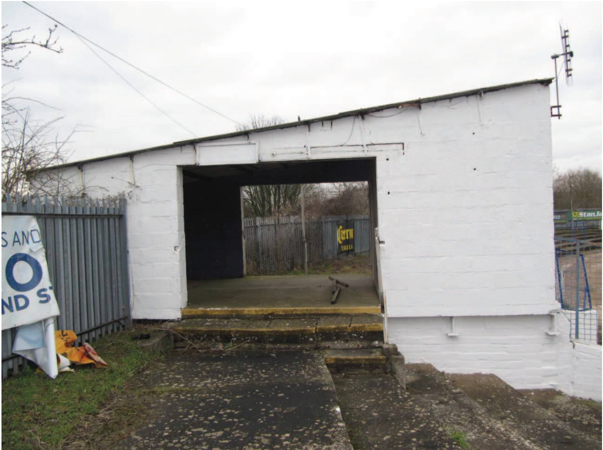
Photograph 21 – terraces to west side of stadium
