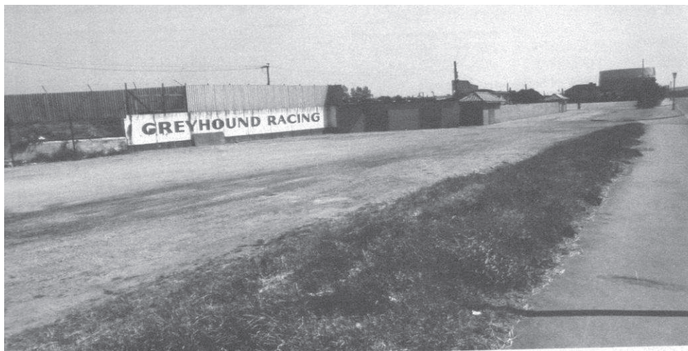
Fig 14: The Stadium from Sandy Lane before the main stand was redeveloped
